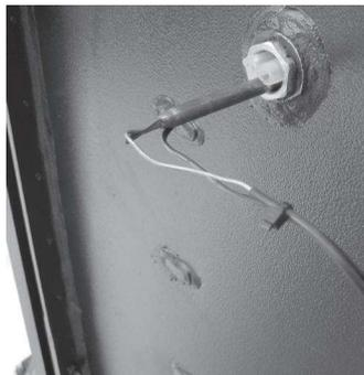
**Water temperature probe:** if the water temperature approaches the blocking temperature (100 °C), the probe requires to interrupt the supply of pellets.
