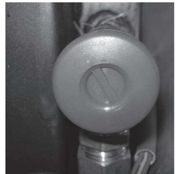
**Safety valve:** this valve acts to prevent over pressurization of the hydraulic system. If the pressure of the thermostove or plant exceeds 2.5 bar it drains the water from the circuit.
